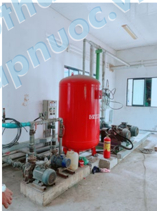
Bình áp VAREM 1000L, 10bar /VAREM pressure tank 1000L, 10bar
